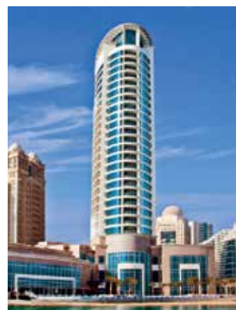
HILTON HOTEL DOHA, QATAR
